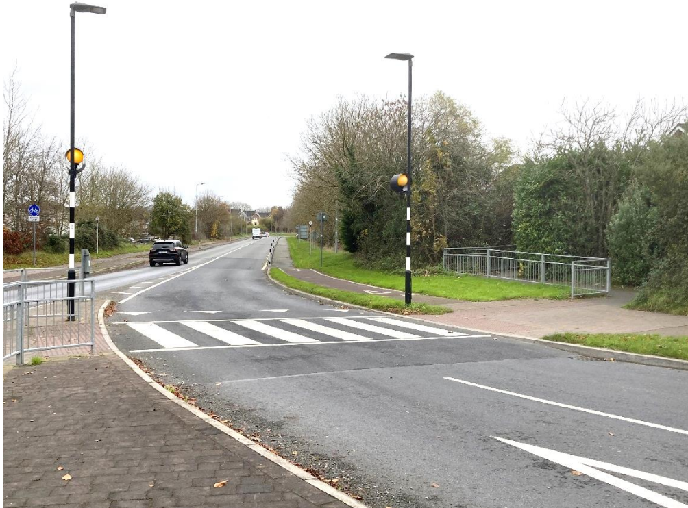
View of cycle lanes either side of R510 from Quinn Cross Roundabout
